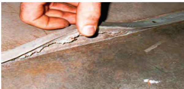
An estimated 80-90% of joint filler installations are performed improperly...
