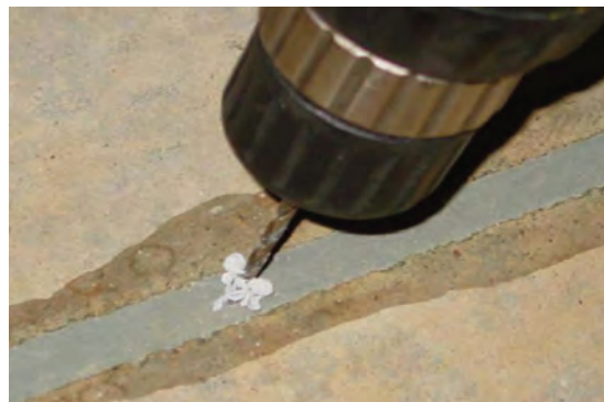
Full joint depth of the filler is easily verified by drilling through the cured filler.
