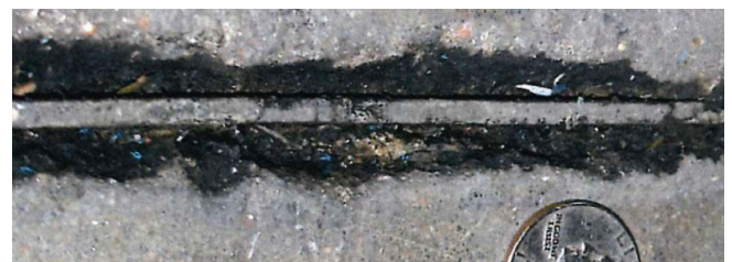
Above: Filler placed over a compressible foam backer rod to reduce material usage. Filler must be placed at full depth to provide joint edge protection.
