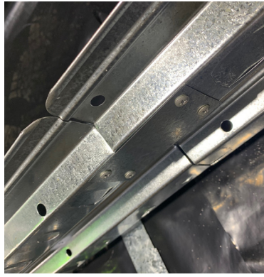
8. Correct use of joiner plane.
