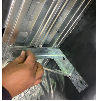
3. Stand up sheet metal and attach brackets to sheetmetal brace.
