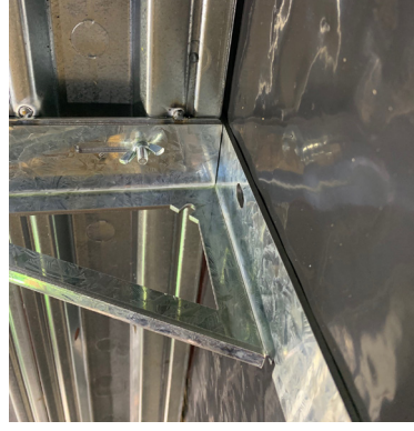
4. Set brackets to lowest position with the sheetmetal sitting on the foot.
